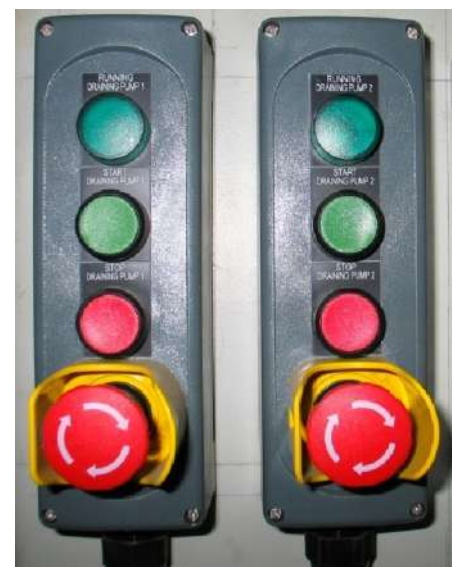
Figure 5-15 Engine Room - Bilge Pumps Remote Control Panels
