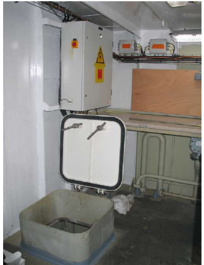
Figure 2-30 Workshop - Storage Room Hatch
