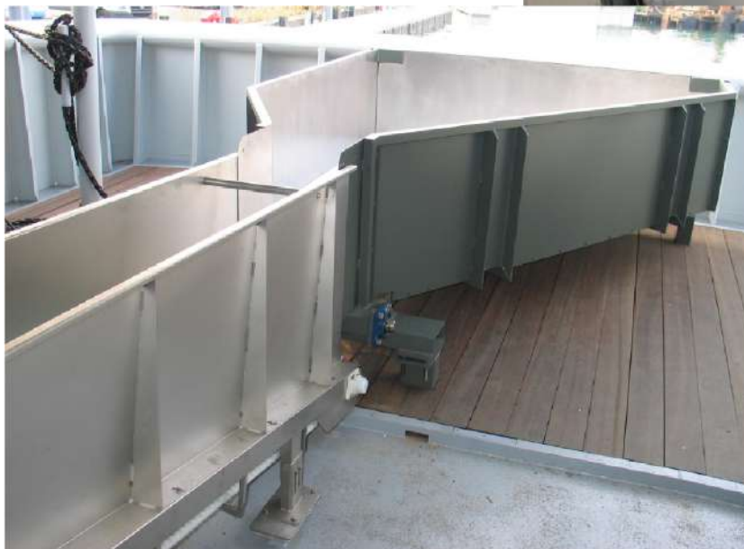
Figure 2-15 Fishing Deck - Fish Conveyor with Unloading Tank
