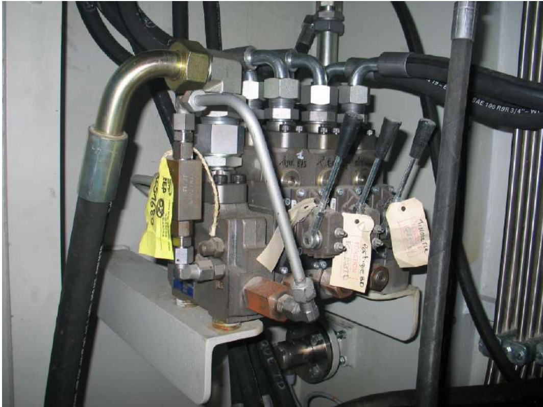
Figure5-49 Store Room - Fishing Gear Hydraulic Distributor
