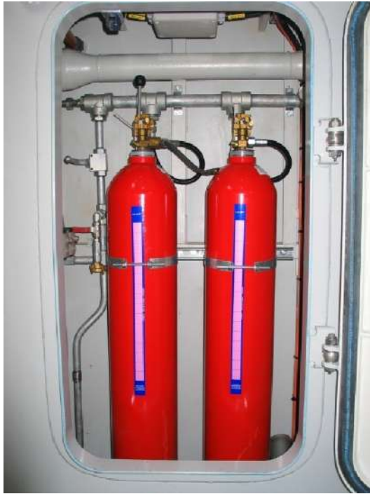
Figure 5-23 CO2 Cylinders 1 and 2
