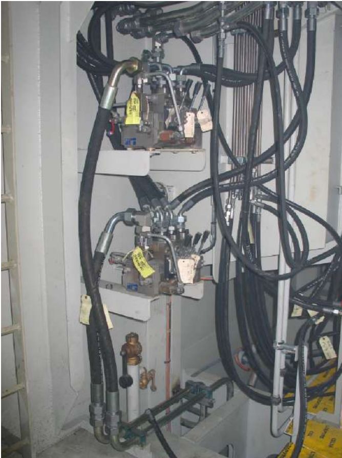
Figure 2-43 Storage Room - Hydraulic Distribution Block for Fishing Gear
