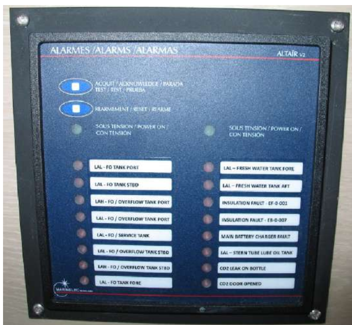
Figure 5-32 Bridge - General Alarm Panel
